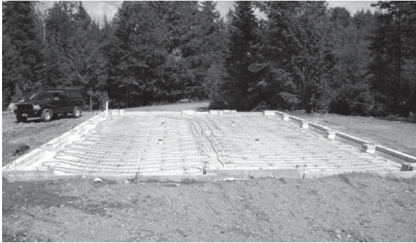
A slab installation using 7/8" PEX tubing, 16" on center
