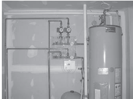
A two zone open system air from a vented attic space and exhausts through the wall with 2" PVC pipe. No chimney is required.
