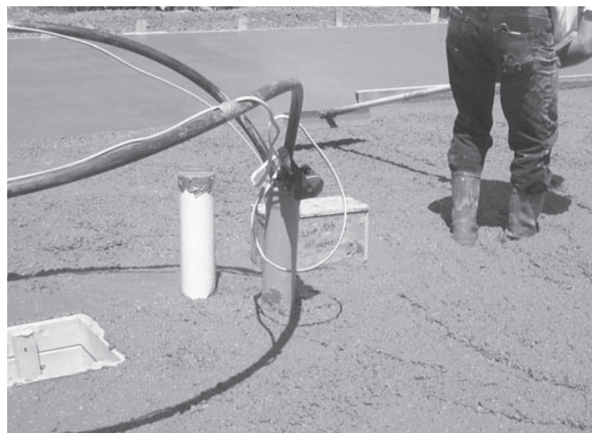
Pouring the slab around the manifold box
