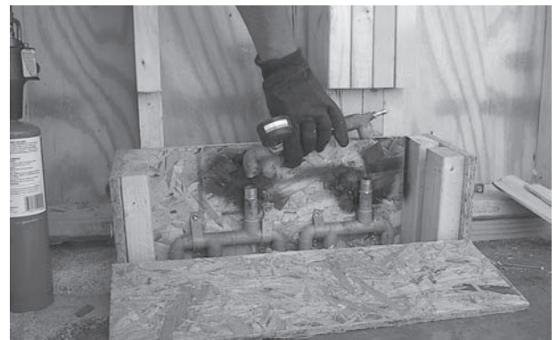
Removing the pressure testing assembly
