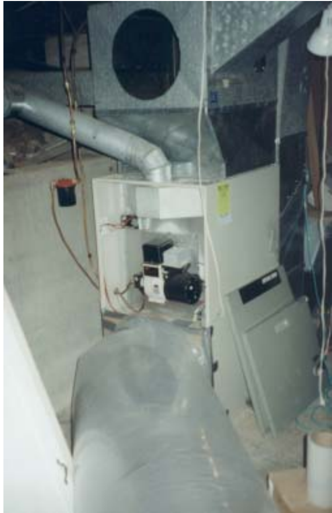
Fig. 2.2. The Aeroseal tubing connection.
