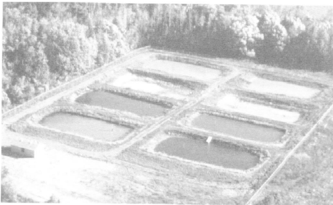
Figure 1. Aquaculture ponds should be fillable, drainable, harvestable, and accessible as needed.
