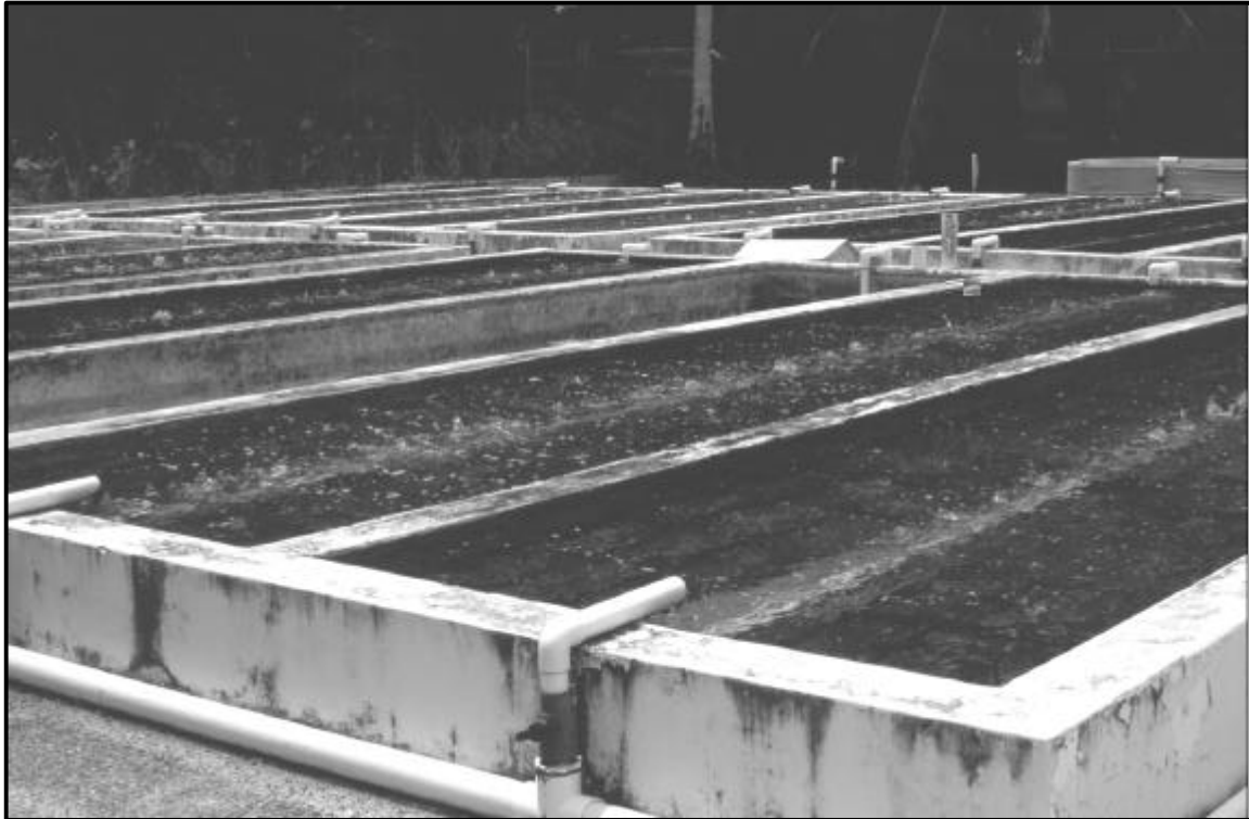
Figure 16. Rectangular concrete raceways at the Palau Mariculture Demonstration Center in the Republic of Belau.
