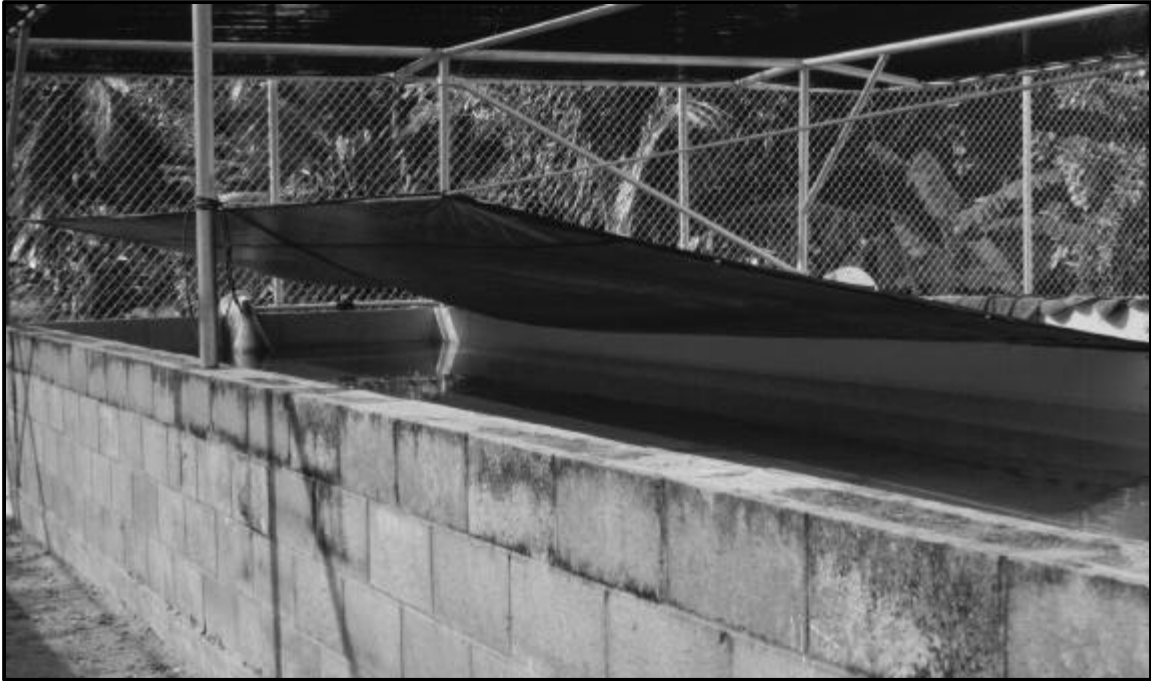
Figure 32. To protect outdoor, static cultures from extreme salinity changes during heavy rainfall a waterproof material, like this shade tarp at the RRE Wau Mariculture facility in Majuro, RMI, is sometimes used to cover all or part of the tank until water flow is started.
