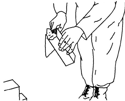
2. SPREADING MORTAR ON BOTH ENDS OF CLOSURE BRICK
