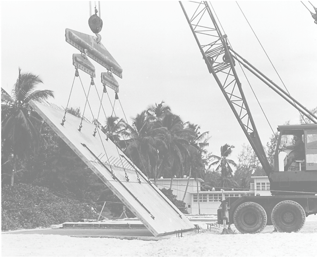
Figure 3-18.—Precast panels being erected by use of crane and spreader bars.
